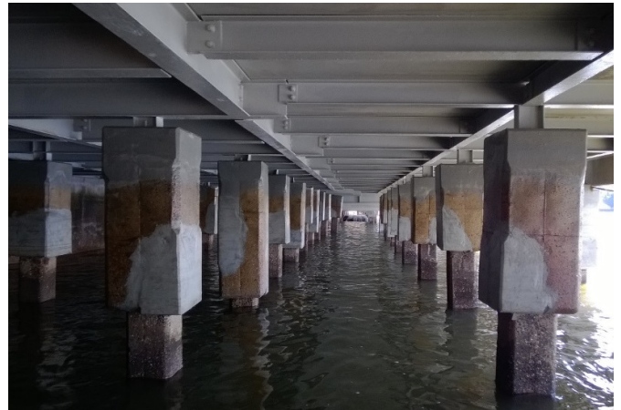
Some of the 92 pile caps that were repaired.
