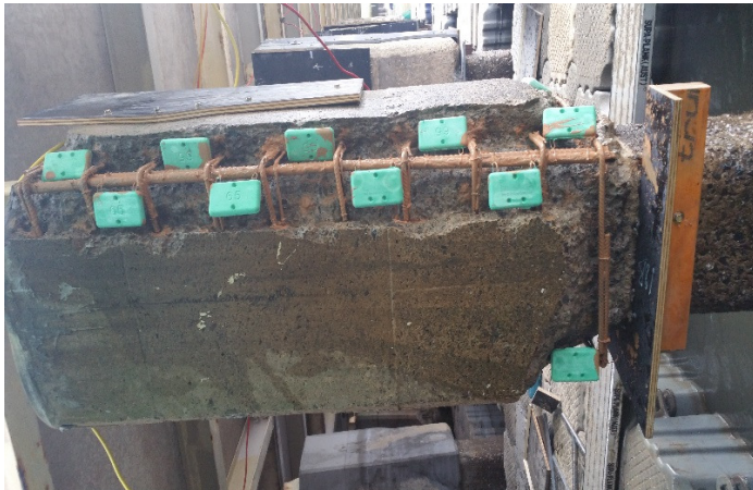
Beam repair preparation and installed MasterProtect 8065 CP sacrificial anodes.
