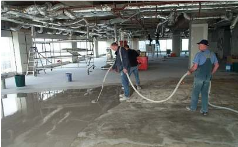
Figure 9 Doing a large area using a pump
