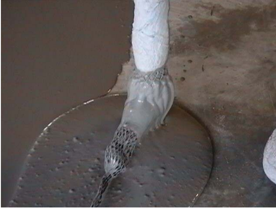
Figure 8 Use of a sock to catch any small lumps coming through the hose
