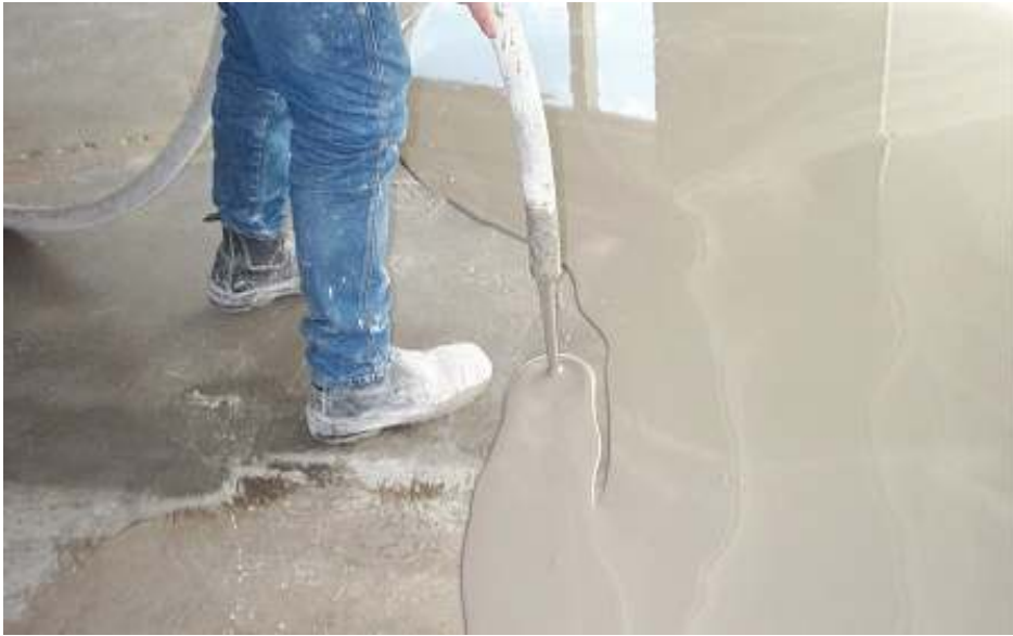
Figure 6 Application from a pump keeping a wet edge
