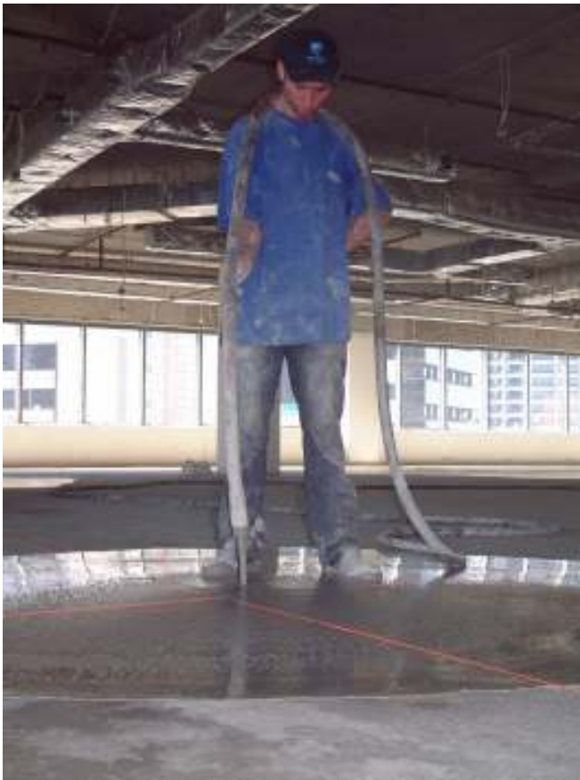
Figure 7 Application from a pump sowing the grid lines to aid in filling the correct depth
