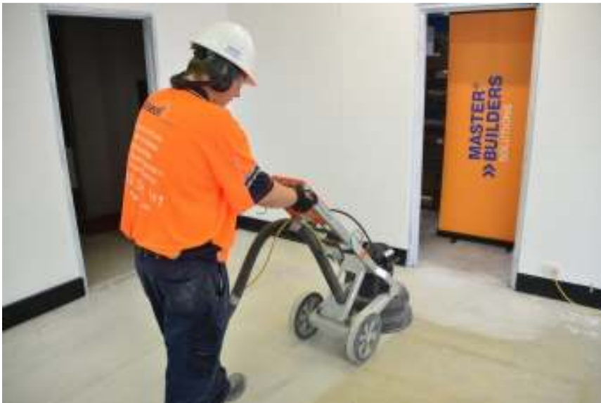
Figure 1 Grinding or shotblasting the preferred methods to prepare the floor
