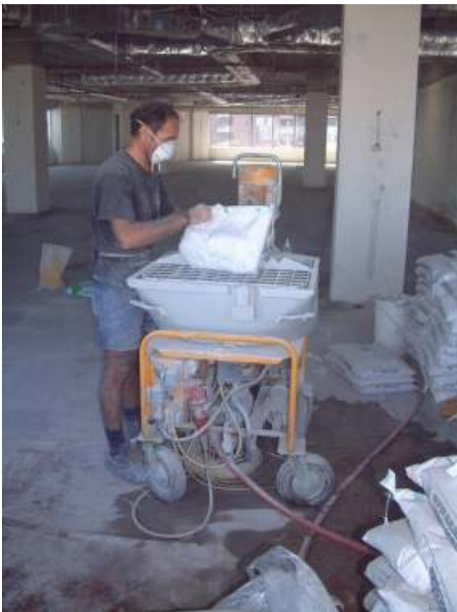
Figure 3 Using the Putzmeister (or other suitable pump to mix continuously)
