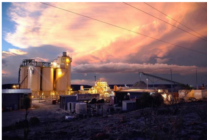
The processing plant at Darlot
