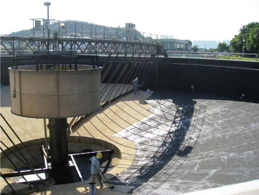
Figure 2 - Application of primer/first coat.
