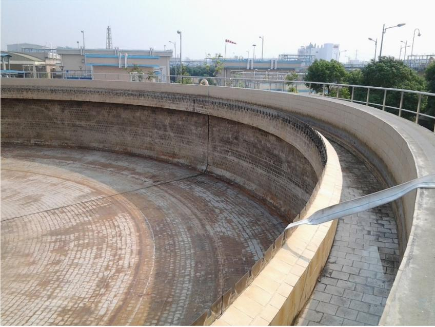
Figure 1 - Cleaned out settlement tank
