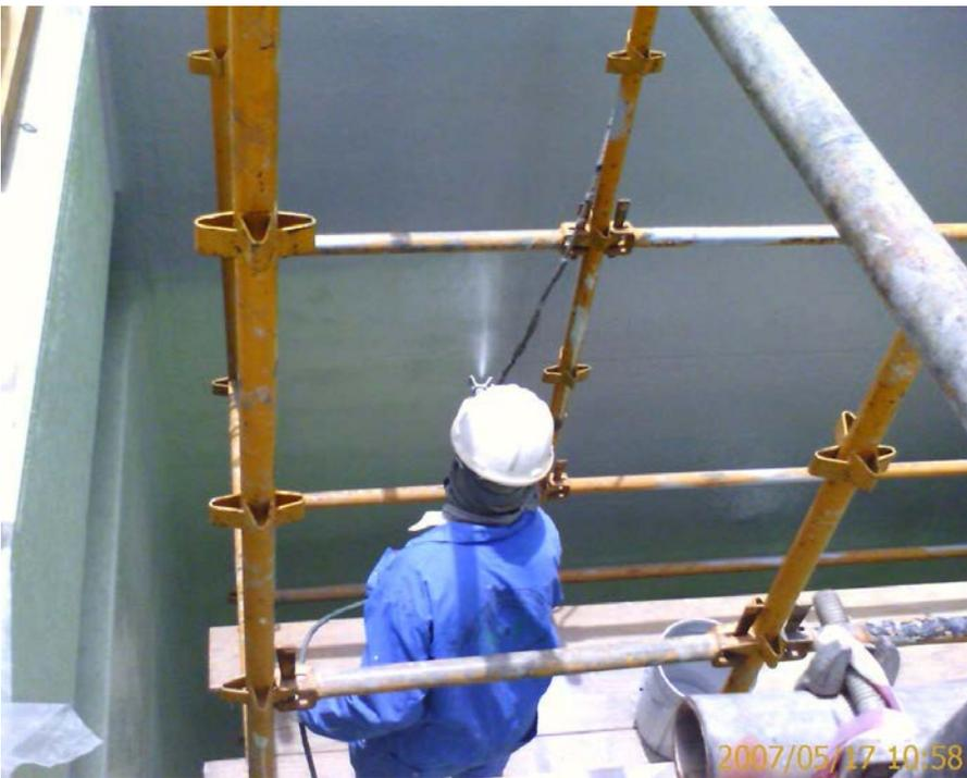
Figure 4 - Spraying final coat on walls.
