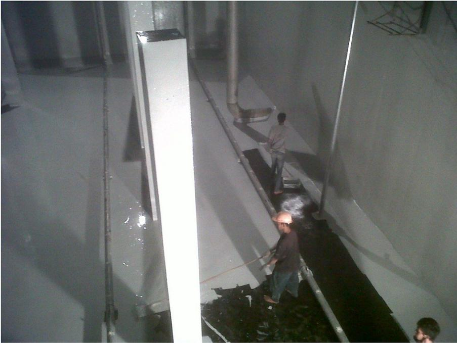
Figure 5 - Applying final coat on floor.
