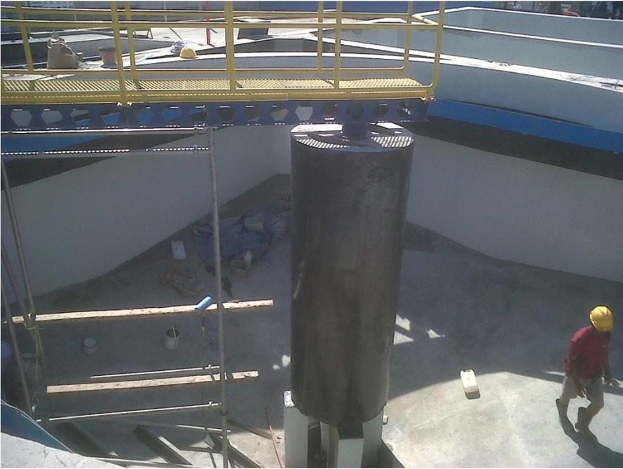
Figure 3 - Preparation of aeration tank.
