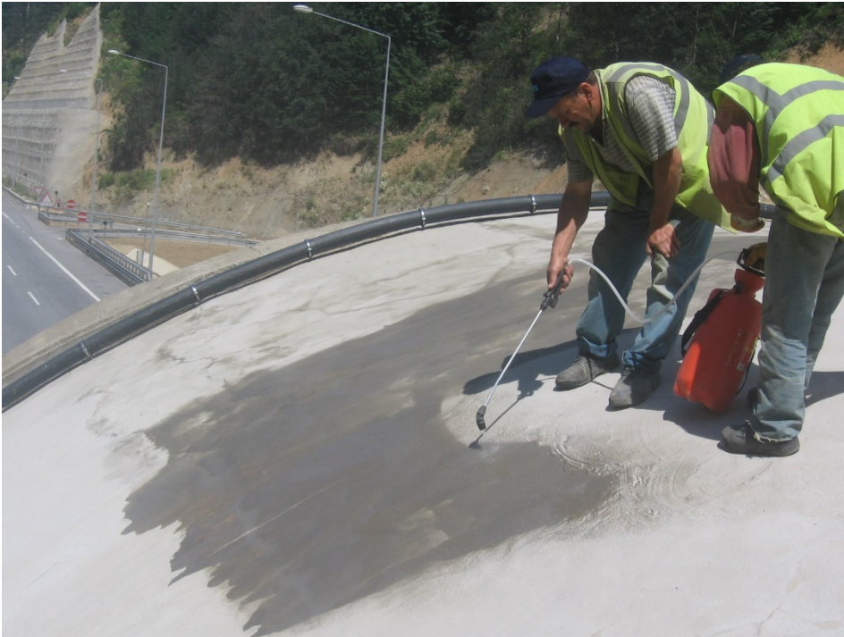
Figure 2 - Application until the material runs
