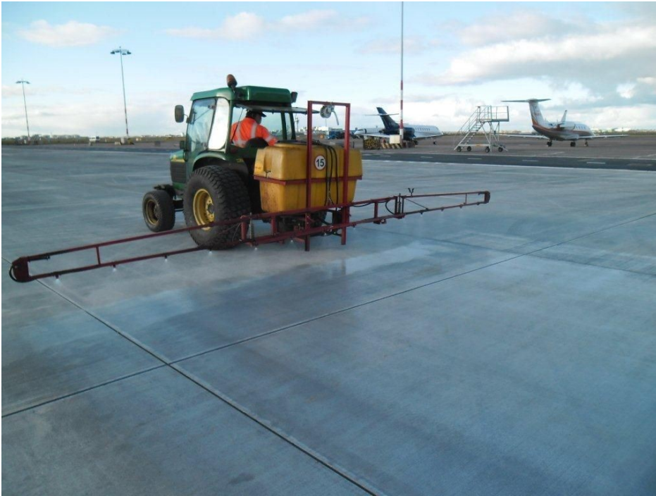
Figure 4 - Spraying large areas with a boom spray for highways or runways.
