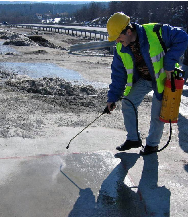
Figure 1 - Applying with low pressure spray
