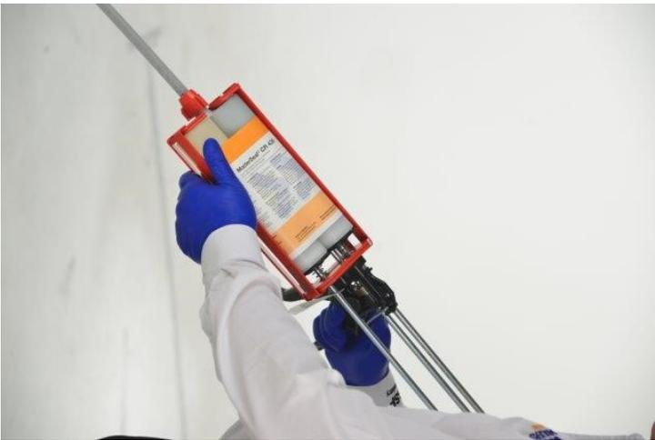
Figure 91414 - Withdraw plunger by releasing the catch plate and remove the cartridge from the gun.
