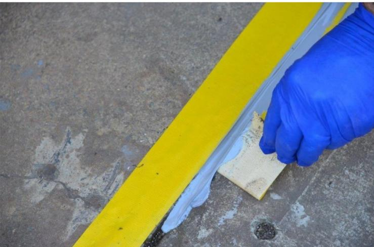
Figure 7212 - Remove tape as soon as tooling is complete
