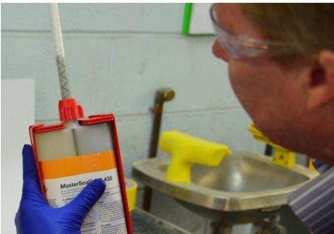
Figure 388 - Hold cartridges vertically to ensure any air in the cartridges is at the top and begin to extrude the material until it starts filling the static mixer. Note the reaction has started and the material in the static mixer will harden if left.
