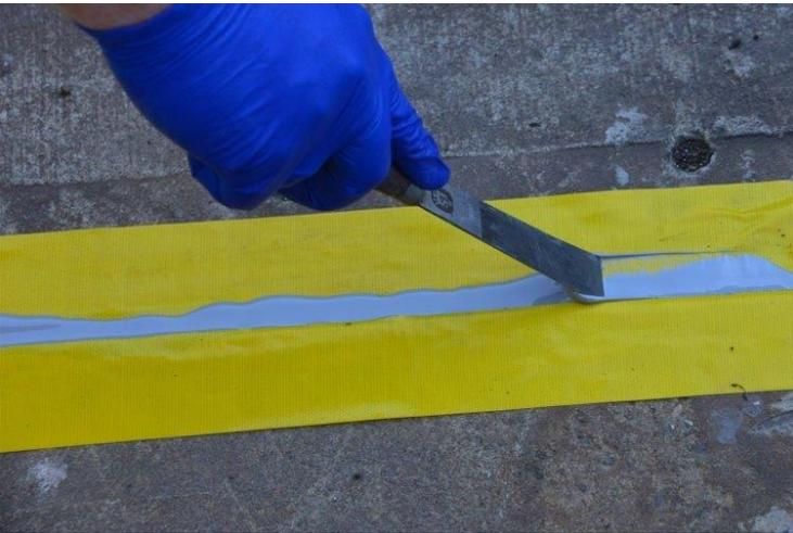
Figure 61111 - Tool off the joint within 3 minutes of gunning the sealant.
