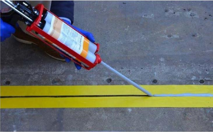
Figure 51010 - Gun material into the joint with smooth presses of the trigger to fill the joint.
