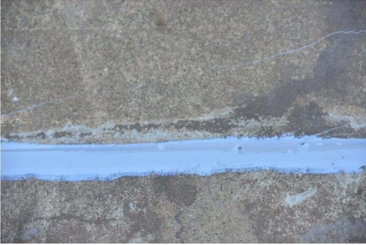
Figure 81313 - Leave joint to cure and return to service after 1 hour
