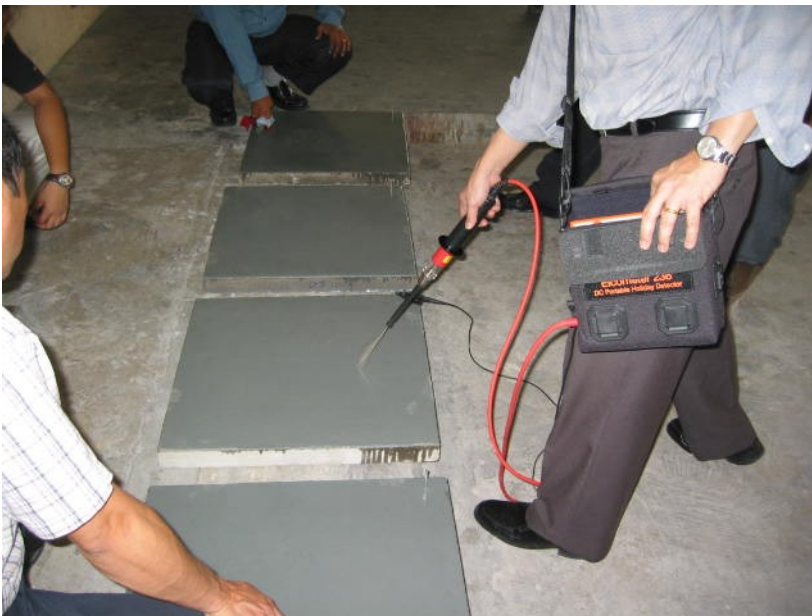
Figure 4 - Holiday testing of membrane
