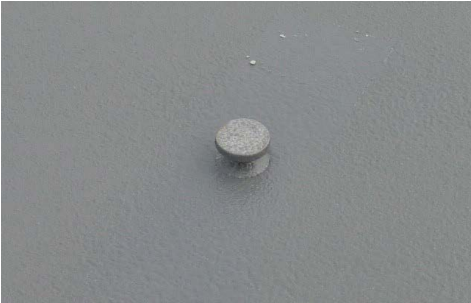
Figure 1 - Adhesion testing dolly adhered to membrane
