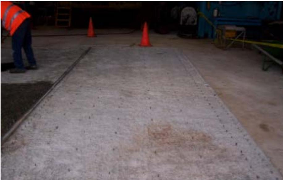
Figure 2 - Long thin section showing extra rows of center pins
