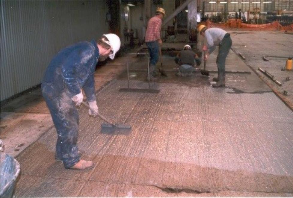
Figure 8 - Applying the MasterEmaco 2525 epoxy bonding agent just in front of the application of the MasterTop 330
