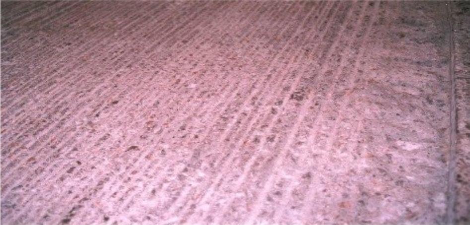
Figure 4 - Well scabbled surface CSP 8 or 9
