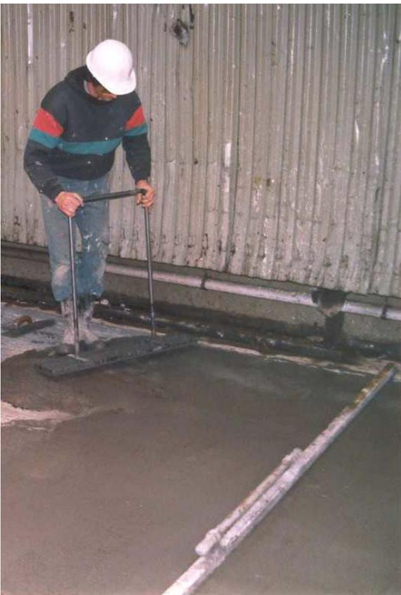
Figure 9 - Using a jitterbug made from a grate to compress and consolidate the MasterTop 330
