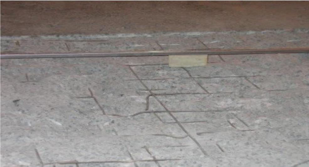
Figure 6 - Set out of section dividers that serve as screed levels and dividers
