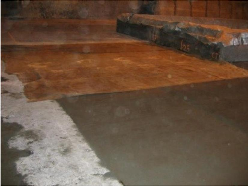
Figure 12 - Curing with wet hessian
