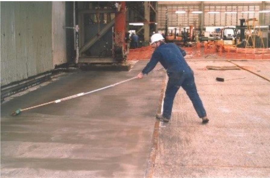
Figure 11 - Applying a broom finish
