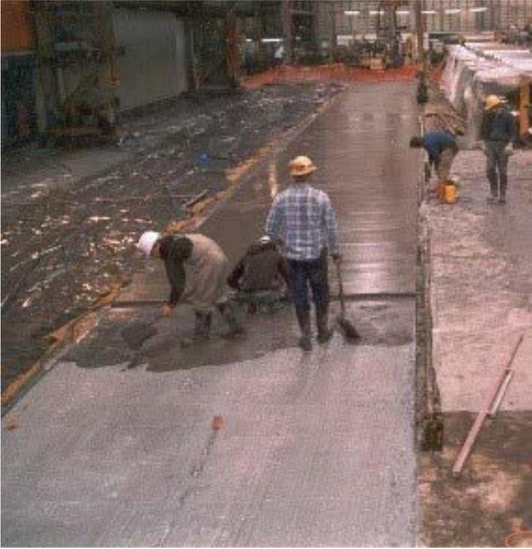
Figure 10 - Mixing station close to the application and multiple mixers to continuously apply
