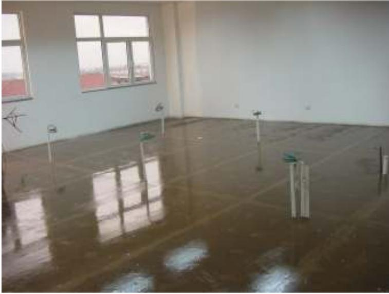
Figure 5 - Primed floor before the application of the bodycoat.
