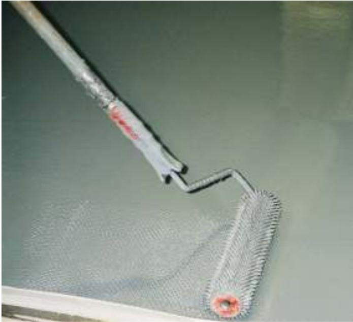
Figure 9 - Spike rolling the applied body coat
