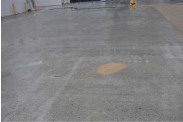
Figure 1 - Prepared floor after shotblasting.
