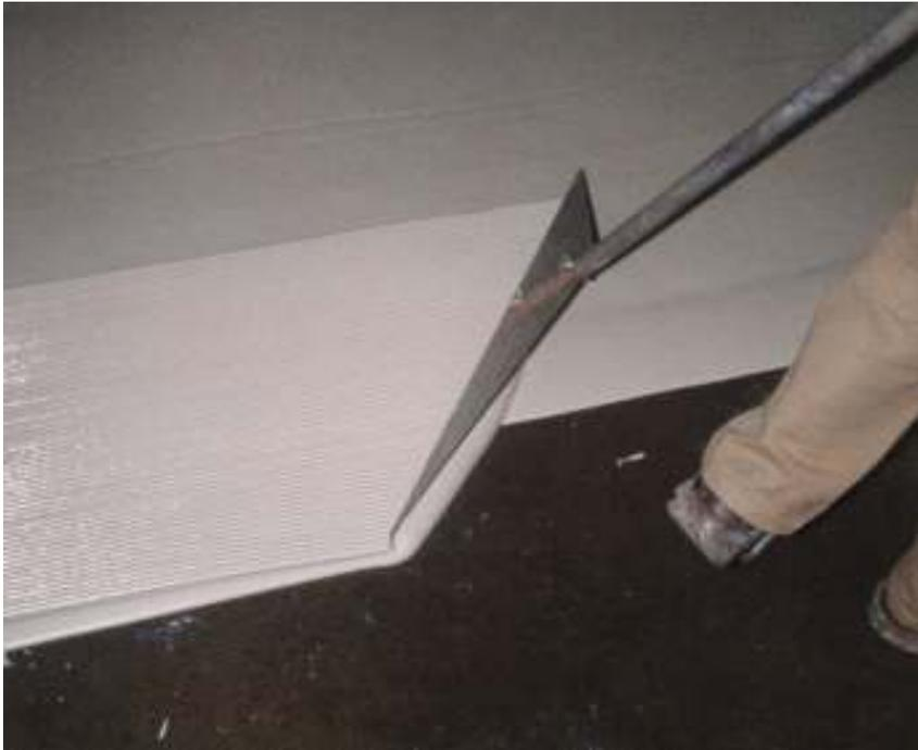
Figure 7 - Applying the body coat by pin rake or notched trowel
