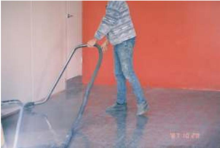
Figure 2 - Vacuuming up the dust after shotblasting.
