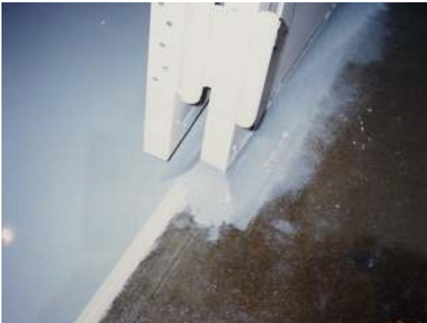
Figure 8 - Cove coated before the application of body coat
