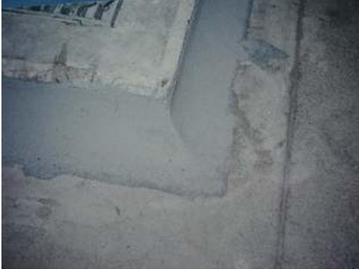
Figure 3 - Prepared cove before application of primer.
