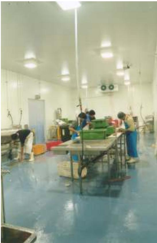
Figure 11 – Non-skid texture of a 2-2.5mm MasterTop 1288 floor
