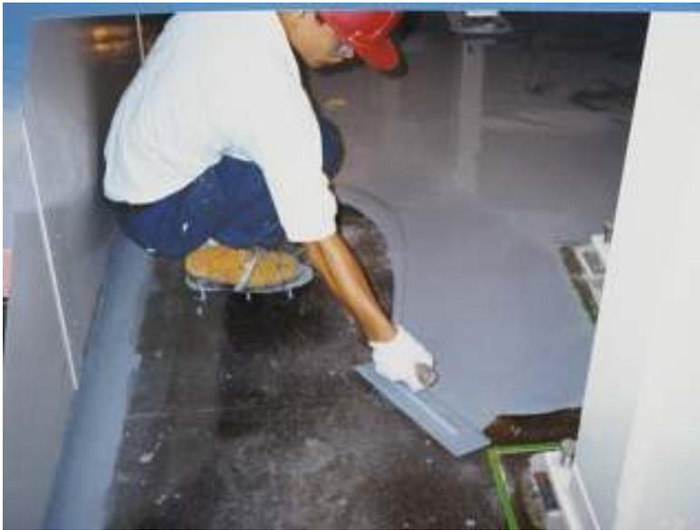
Figure 6 - Applying the body coat by trowel
