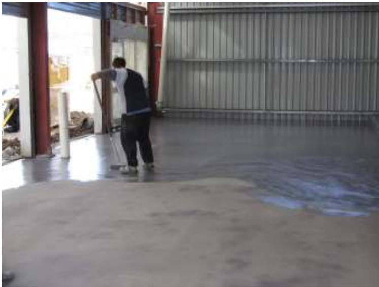
Figure 4 - Priming the floor.
