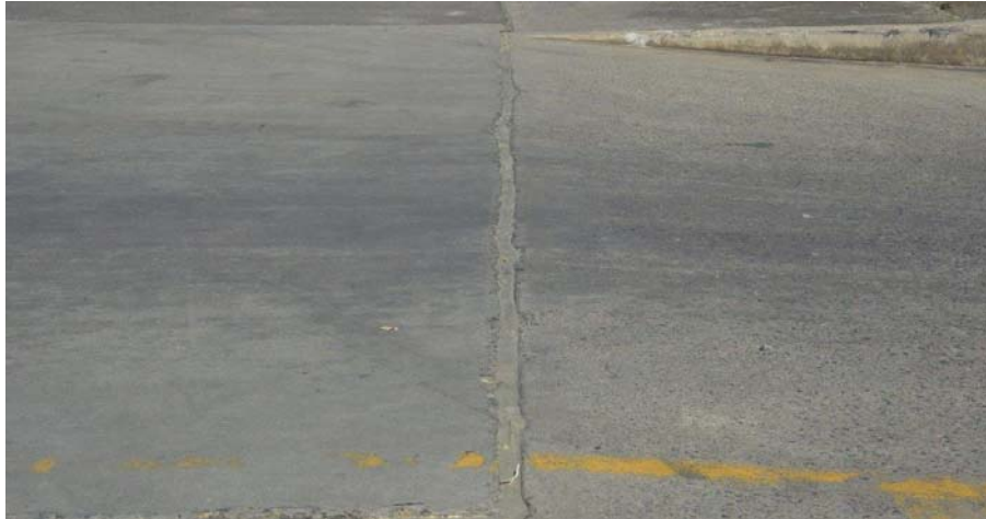
Photo: The repaired joint outside BASF Seven Hills warehouse driveway
