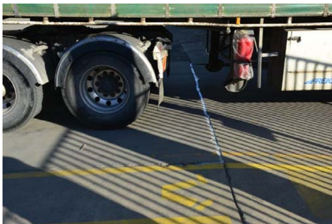
Photo: Traffic moved over the joint within 15 minutes of application
