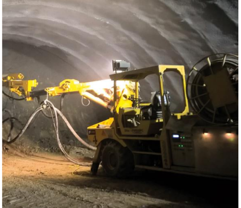
Barcelona (Spain): Olesa Twin Tunnel
