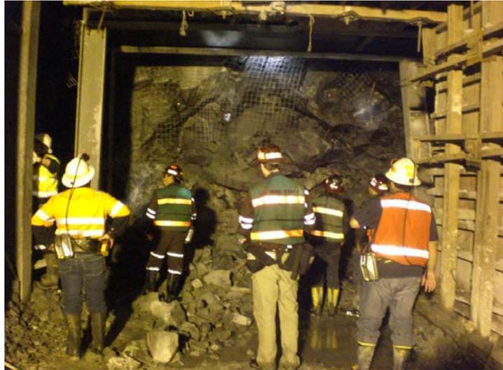
Ground collapse at Freeport underground mine production area. Location at panel 5, Deep Ore Zone underground mine.
