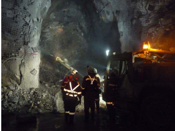
Sprayed concrete (shotcrete) trial at Kencana and Toguraci underground mine, Gosowong gold project
