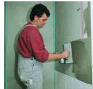
6. When the waterproofing MasterTile WP 668 has cured tiles can be laid.
