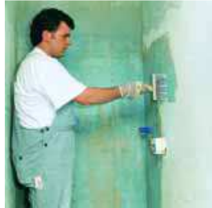
1. Priming: Prime absorbent mineral or gypsum-based substrates and plaster boards with MasterTile P 302 .
