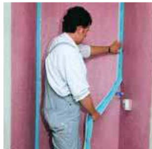
3. Fix MasterTile WP Tape with MasterTile WP 668 (red) in corner joints and floor/wall junctions.
