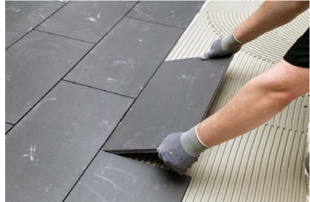
Secure laying of tiles with MasterTile 434
