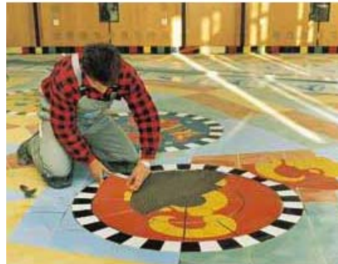
Secure laying of tiles with Mastertile FLX 23
