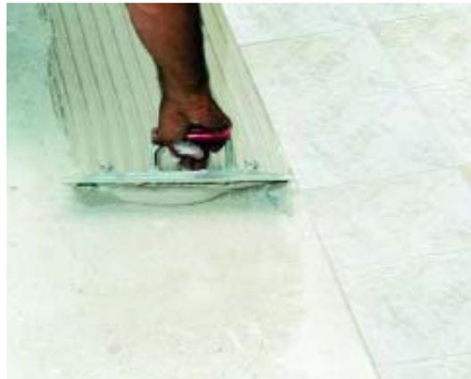
**MasterTile NTS 26 Rapid** is a workable medium-bed mortar easy to apply.
