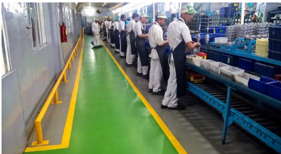
Ucrete flooring installed in the Engine Assembly Shop, Atlas Honda Karachi Plant
