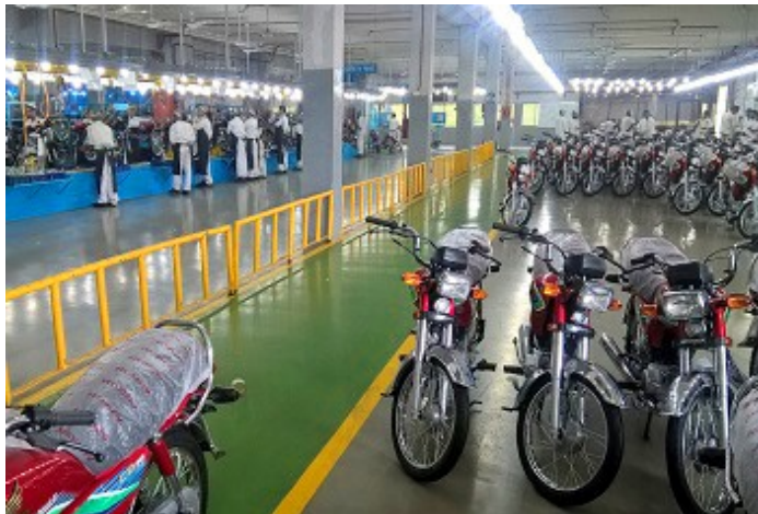
Ucrete flooring installed in motorcycle assembly line, Atlas Honda Karachi Plant
