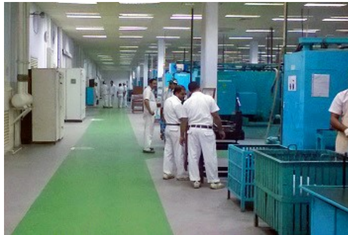
Ucrete flooring installed in hi-tech machine shop, Atlas Honda Lahore Plant
