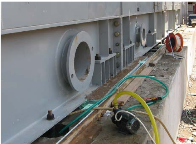
Figure 1. Saturating and draining the excessive water in the anchor holes of the turbine foundation prior to grouting.
