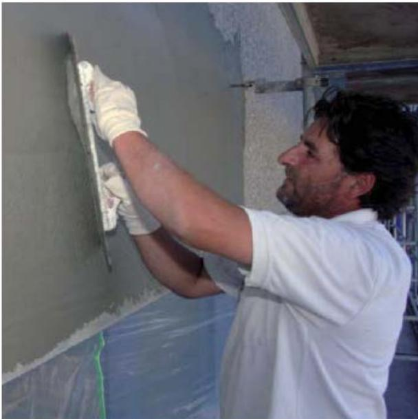
MasterEmaco N 5100 is a ready-to-use material, containing special cements, optimally matched by grain size sand, a mixture of polymer additives, and a polymer fiber.
