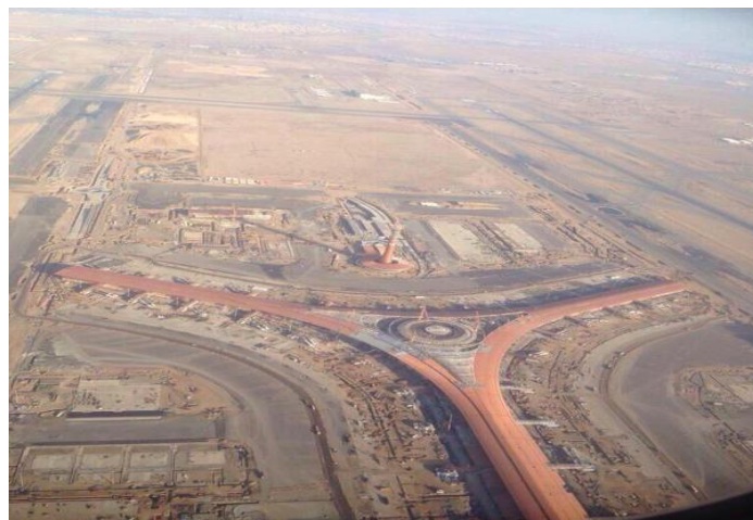
Our reference in western province (Kingdom of Saudi Arabia): KAIA Picture Source: construction site.
