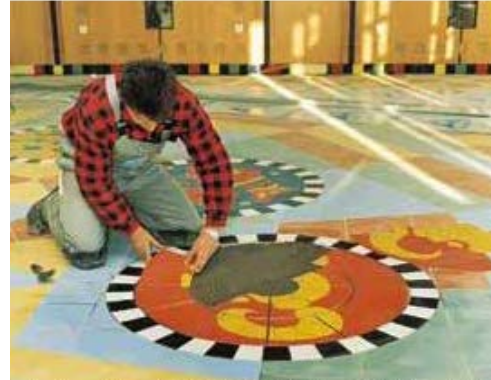
Secure laying of tiles with Mastertile 21
