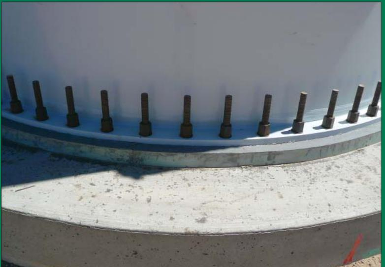
Grout and concrete work together to create a durable foundation for a wind turbine. To achieve long-term performance of wind turbine towers, quality grout materials and knowledgeable installation are a must.
