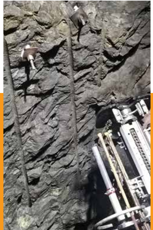
Self-drilling anchor with MasterRoc RBA 380
