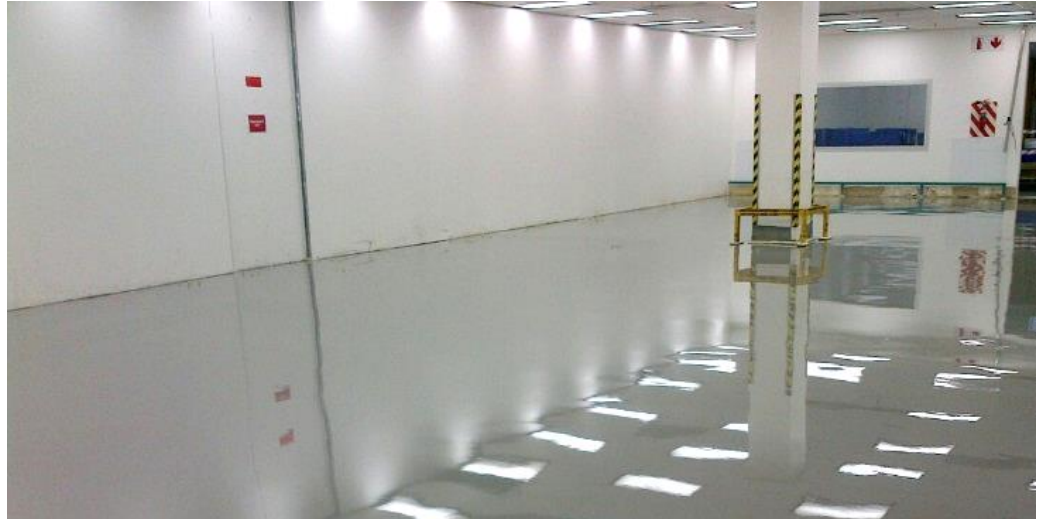
Our reference in Aeroton (South Africa): Adcock Ingram Critical Care facility
