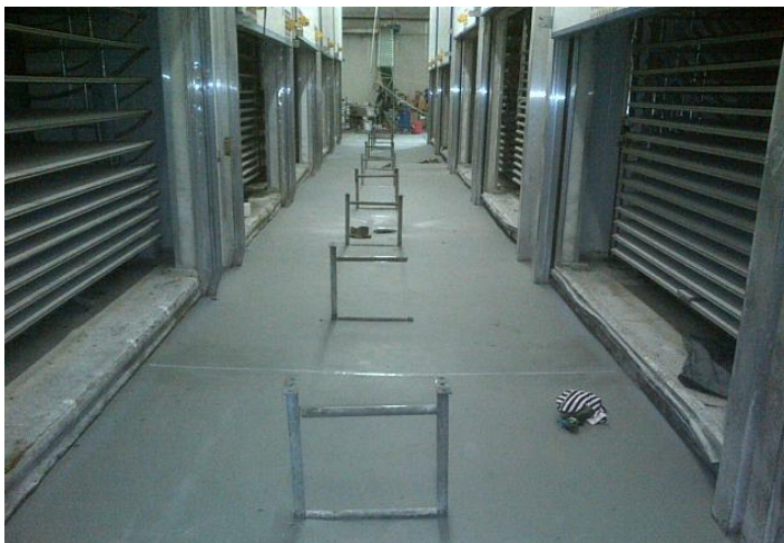
Our reference in Aeroton (South Africa): Adcock Ingram Critical Care facility
