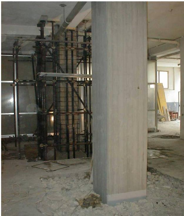
It is applied by casting also into formwork on macroscopically roughened concrete (surface irregularity of approx. 5 mm) for a repair thickness between 6 and 10 cm inclusive.
