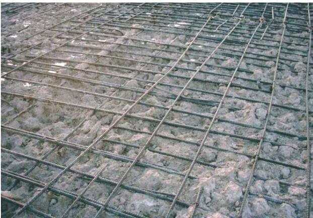
The surface of the concrete substrate must be macroscopically rough (surface irregularity approx. 5 mm deep) to obtain maximum bond between the substrate and the repair material. The macro-roughness is indispensable for the restrained expansion mechanism, which is essential for the success of shrinkage compensated cementitious mixes.
