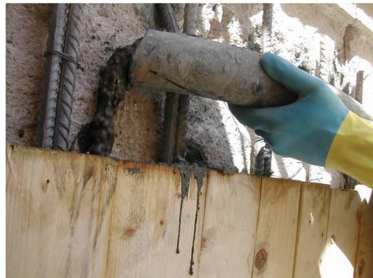
Its particular rheology means it can compact without requiring vibration and can flow even in structures that are heavily reinforced or have a complex shape.
