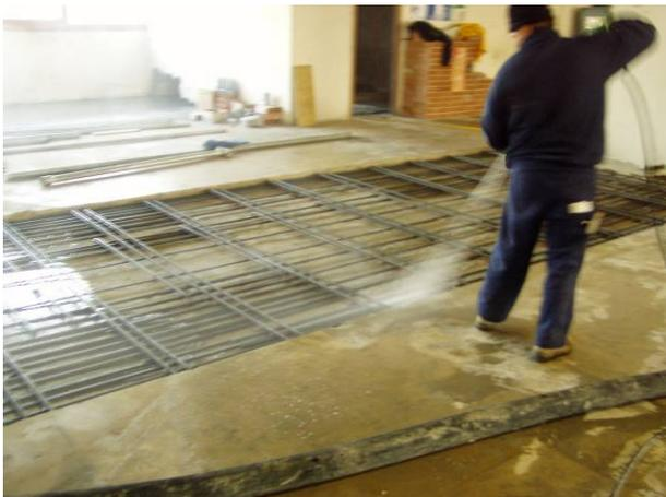
Cleaning and saturation of the surfaces are essential to obtain high values of adherence between base and filler material.
