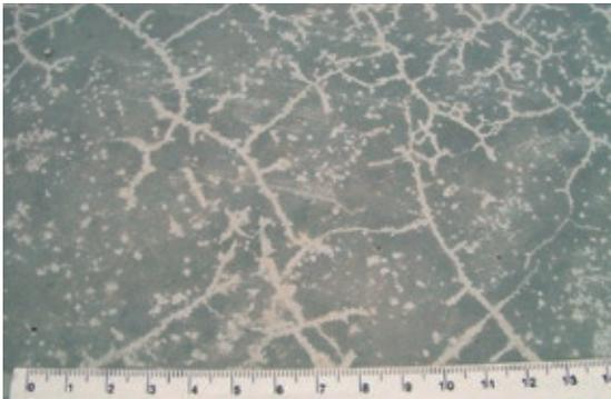
Early age cracks by drying shrinkage
