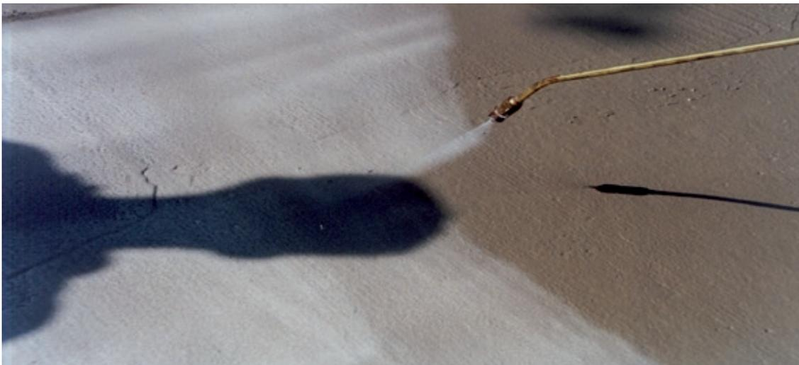
MasterKure application on construction site after placing the concrete
