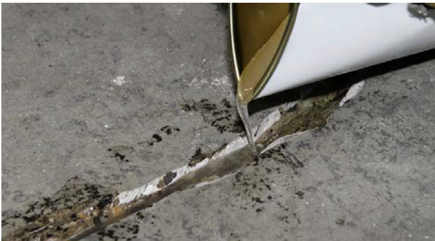
Figura 4. Turnarea MasterInject 1360 direct in fisura deschisa in forma de V
