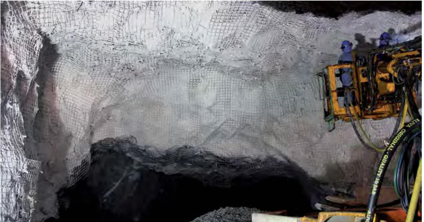
In hard rock mining, oxidation can affect weak strata, causing rock slabbing and roof and wall degradation. Effective surface support and the protection of rock and strata against weathering are critical to the safety and efficiency of any mining operation.
