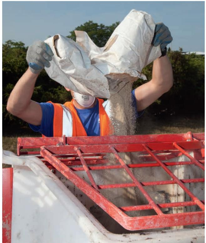
**FIGURE 1.** The aggregate component of a polymer grout acts as a heat sink to absorb the heat created by the exothermic reaction between the epoxy resin and the amine hardener
