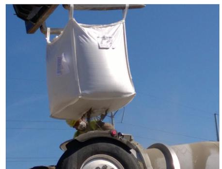
As the wind direction can affect this operation, park the transit truck so the worker is not facing the prevailing wind. Take care that no vehicles or structures are downwind. Success has been achieved mixing between 2 and 4 bulk bags per batch. When mixing 3 or 4 bags at a time, the remainder of the mix water should be added between bags 2 and 3.
