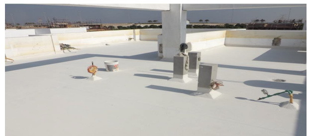
Accessible screed roof protected by MasterSeal 550 K
