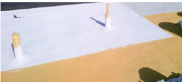
PU foam protected with MasterSeal 550 K
