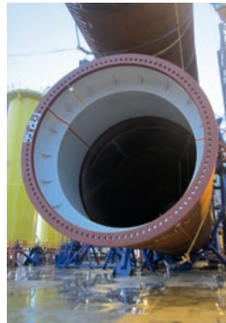
Monopile on deck
